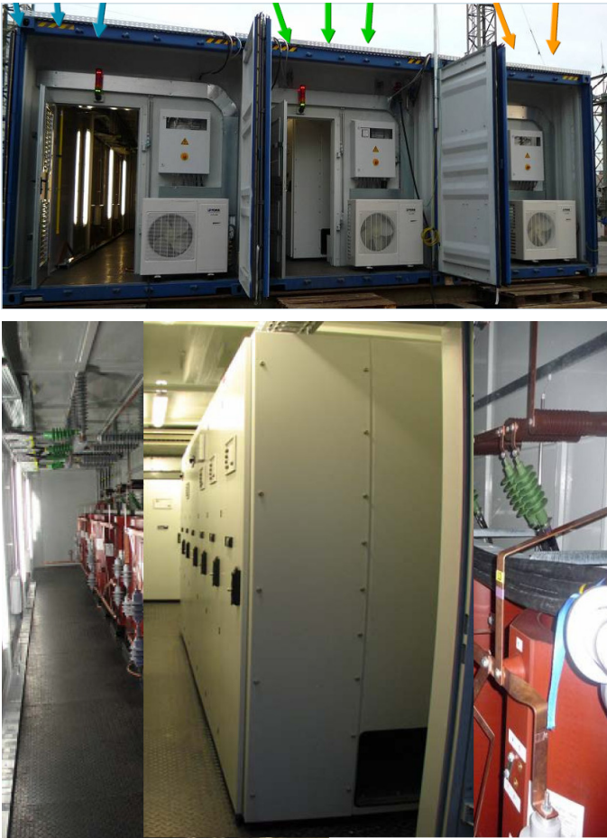
Figure 9. Photographs of a sag generator
